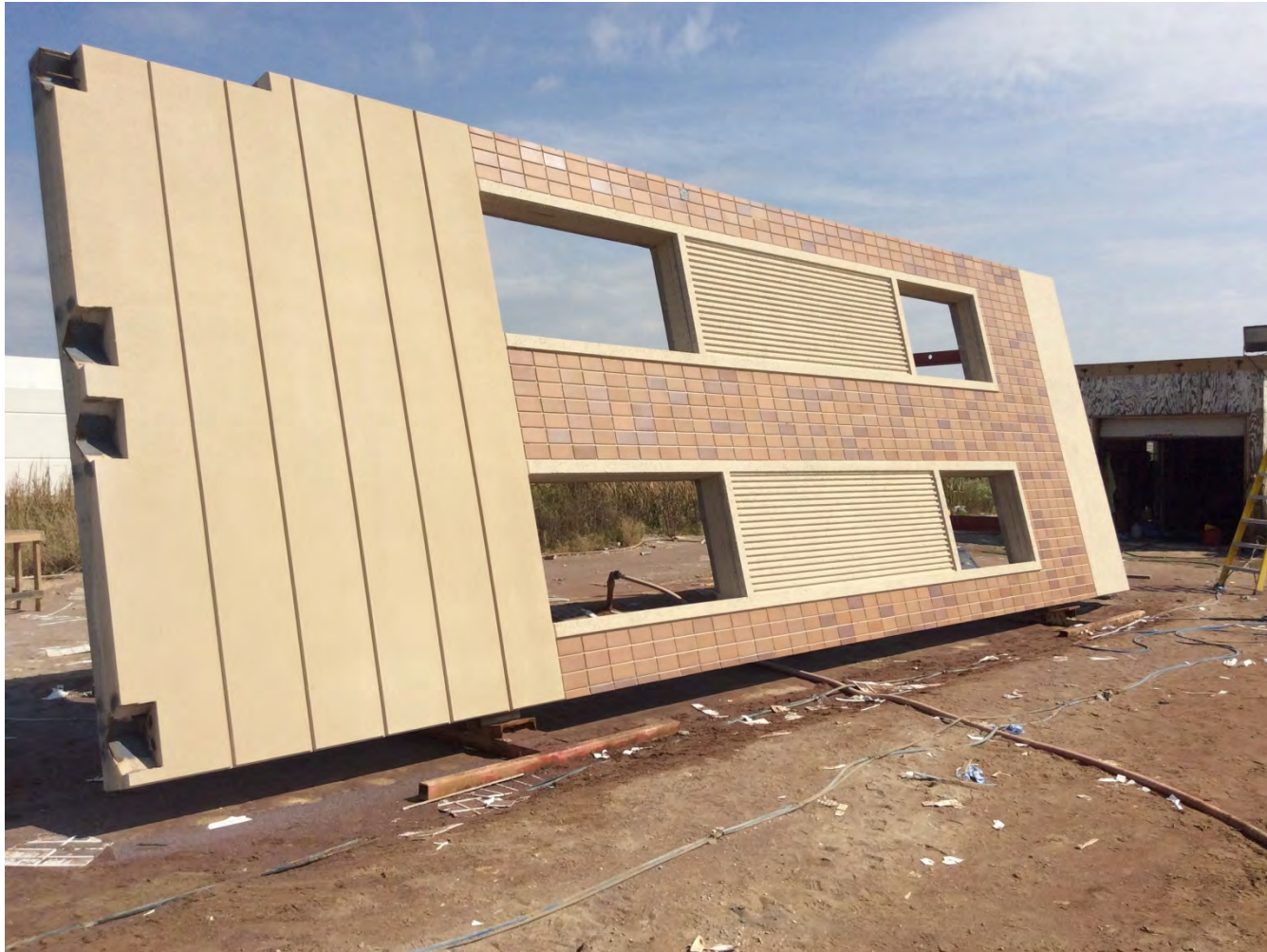
Panel #11W-069 North Elevation Alongside East Stairwell
