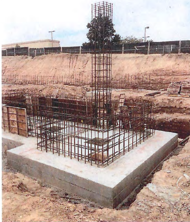
Elevator Pit Foundations
