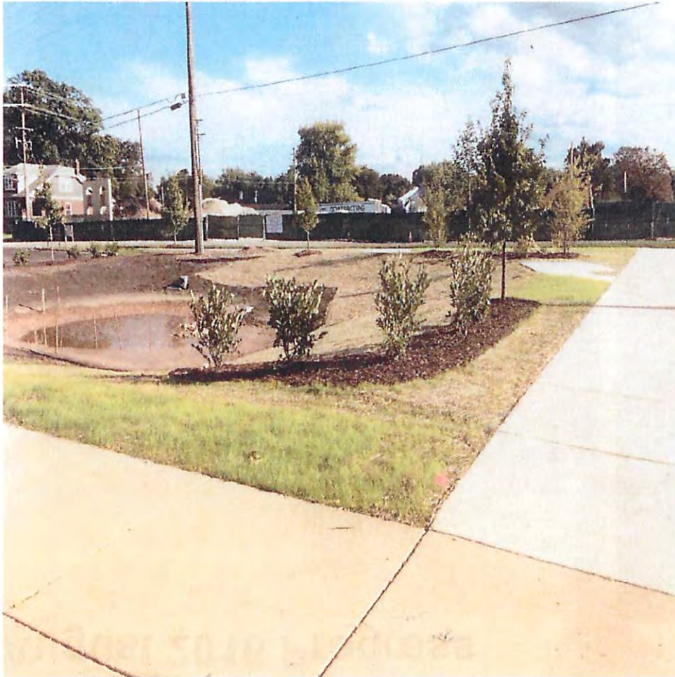
Detention Basin At Exchange & Locust Intersection
