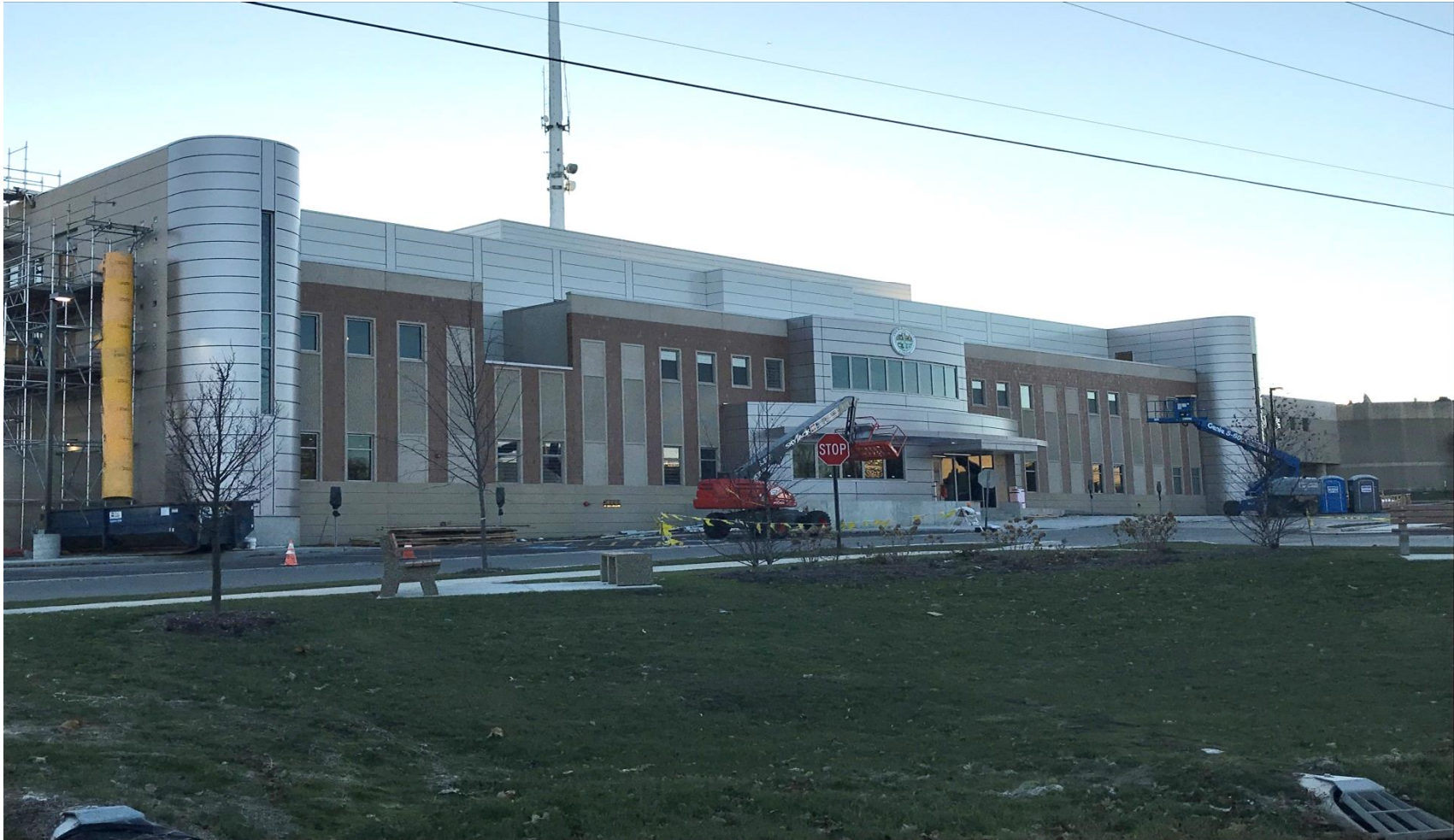
North Elevation Progress
