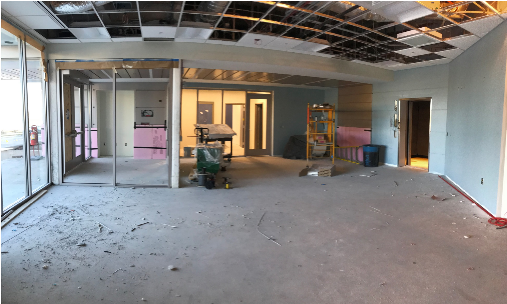
Front Lobby Progress
