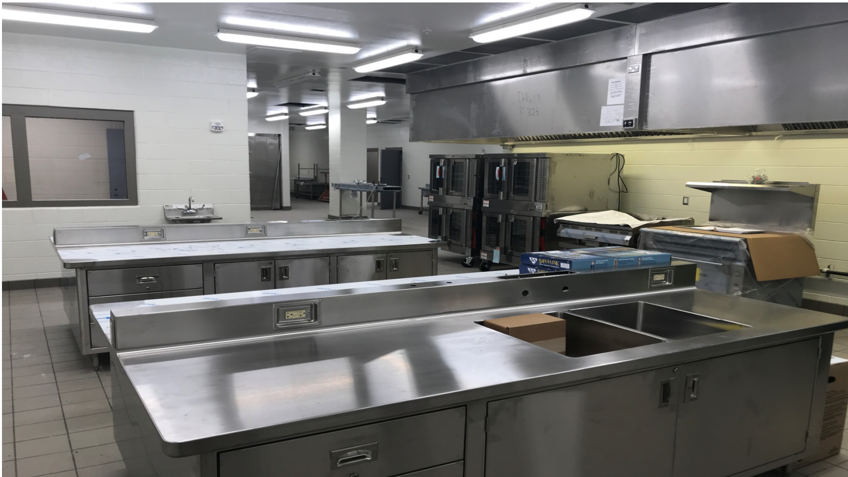
Kitchen Equipment Installation
