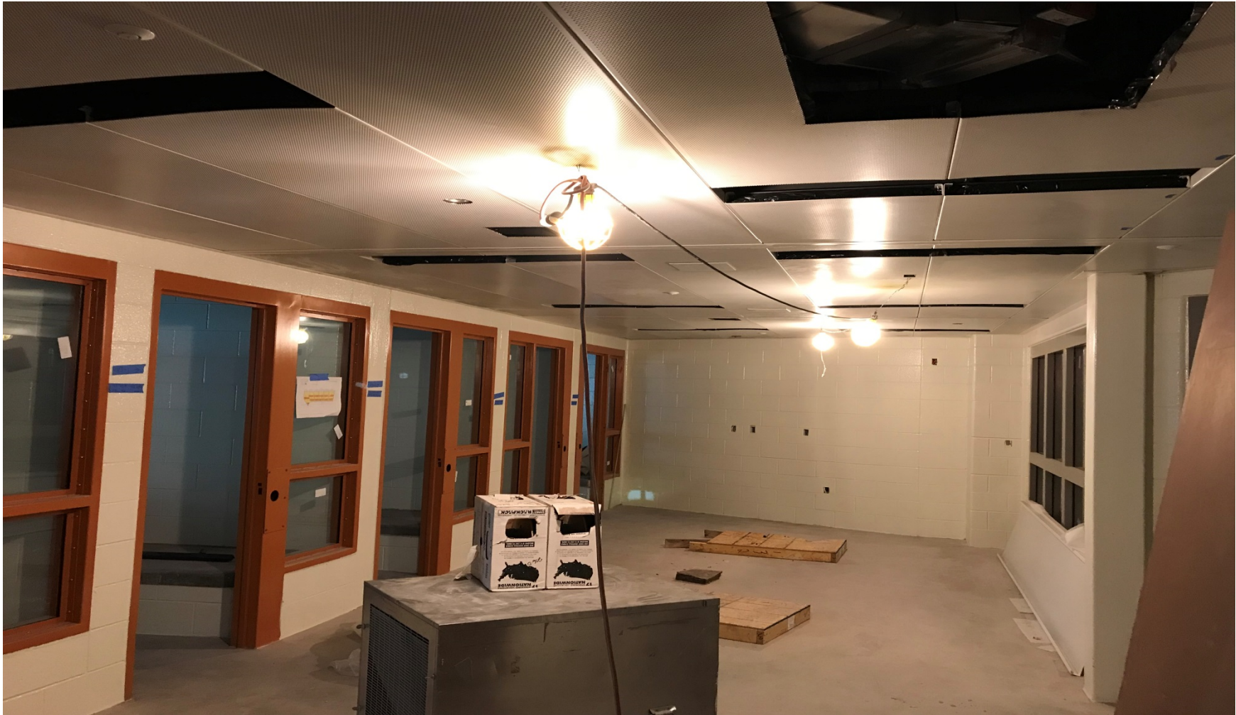
2 nd Floor Dayroom N Progress
