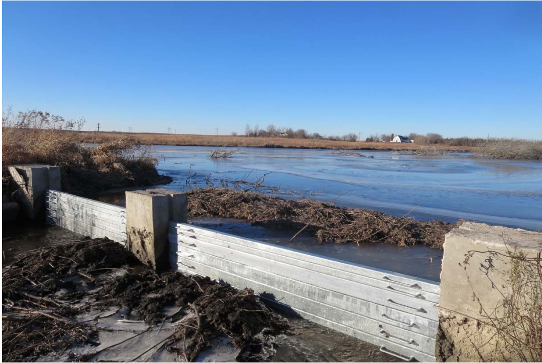
Half of a beaver dam stands behind the shiny new steel gates in the Phase 2 marsh at Afton.
