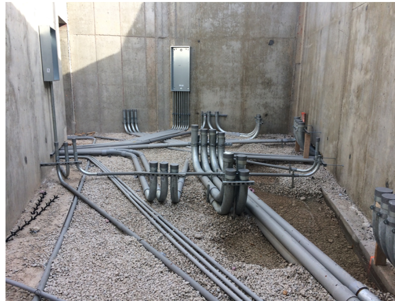
Electrical Room Underslab Rough In (Pictured Above)
