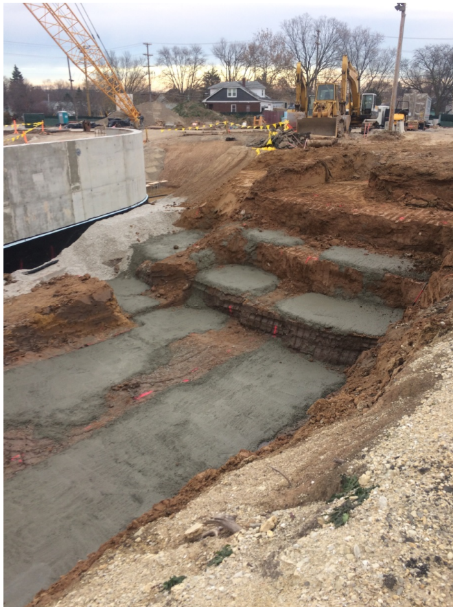
Concrete Mudmat For Loading Dock Foundations (Pictured Left)
