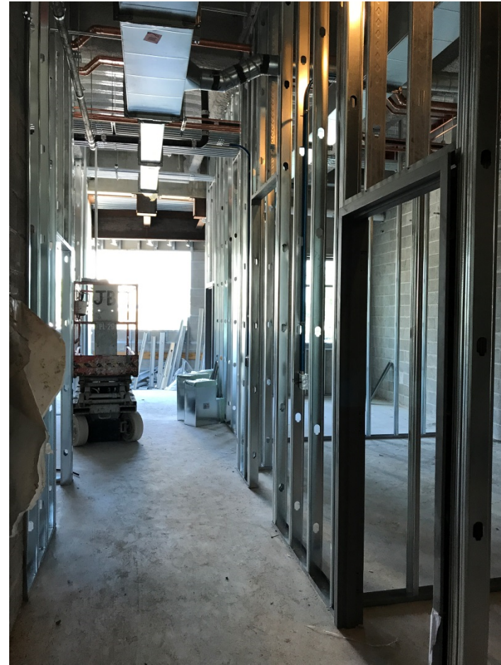
1 st Floor West Painting & Overhead Rough In (Left) and Staff Area Framing
