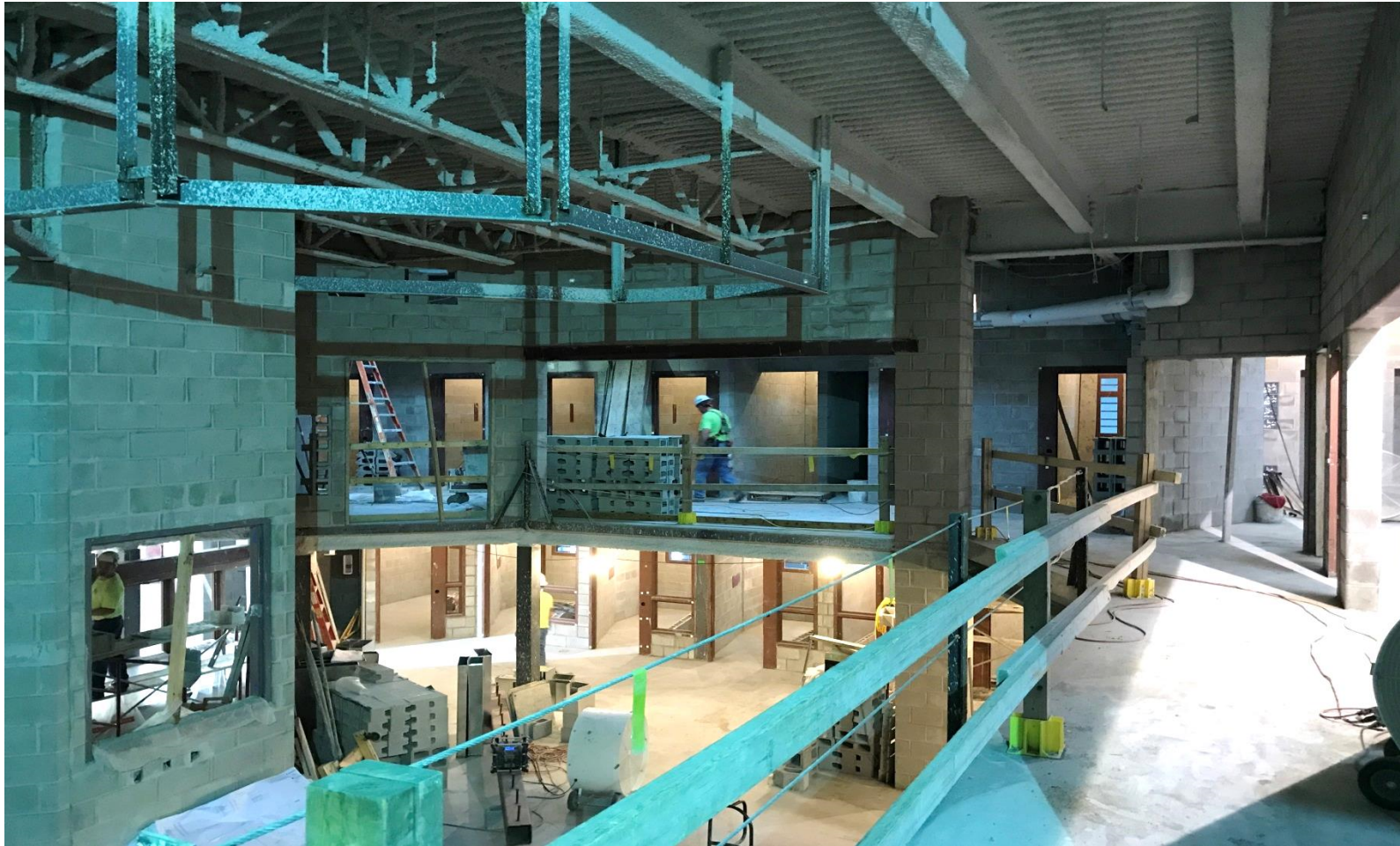
3 rd Floor Mezzanine Area Looking Across Control Platform
