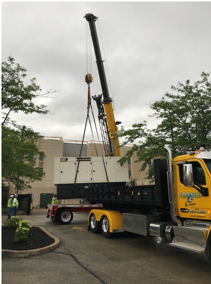
Twin 600KW Generator Arrival & Installation
