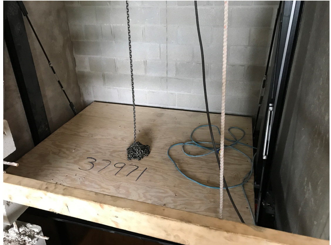
Elevator E-1 (Public Car) Installation
