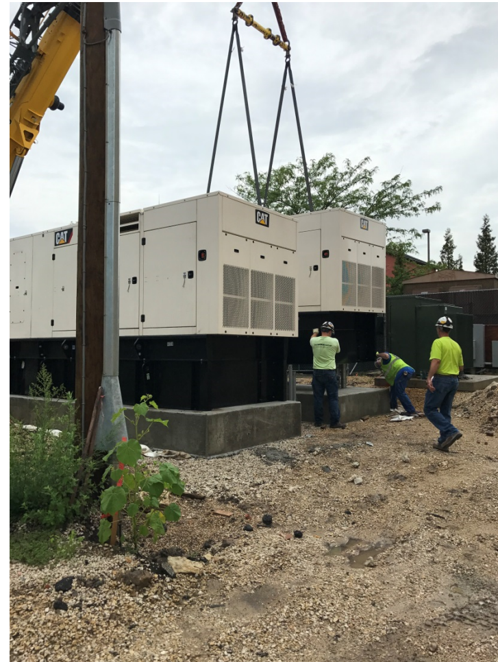
Twin 600KW Generator Arrival & Installation
