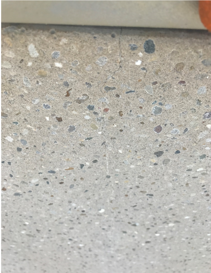
Hairline Cracking in Precast
