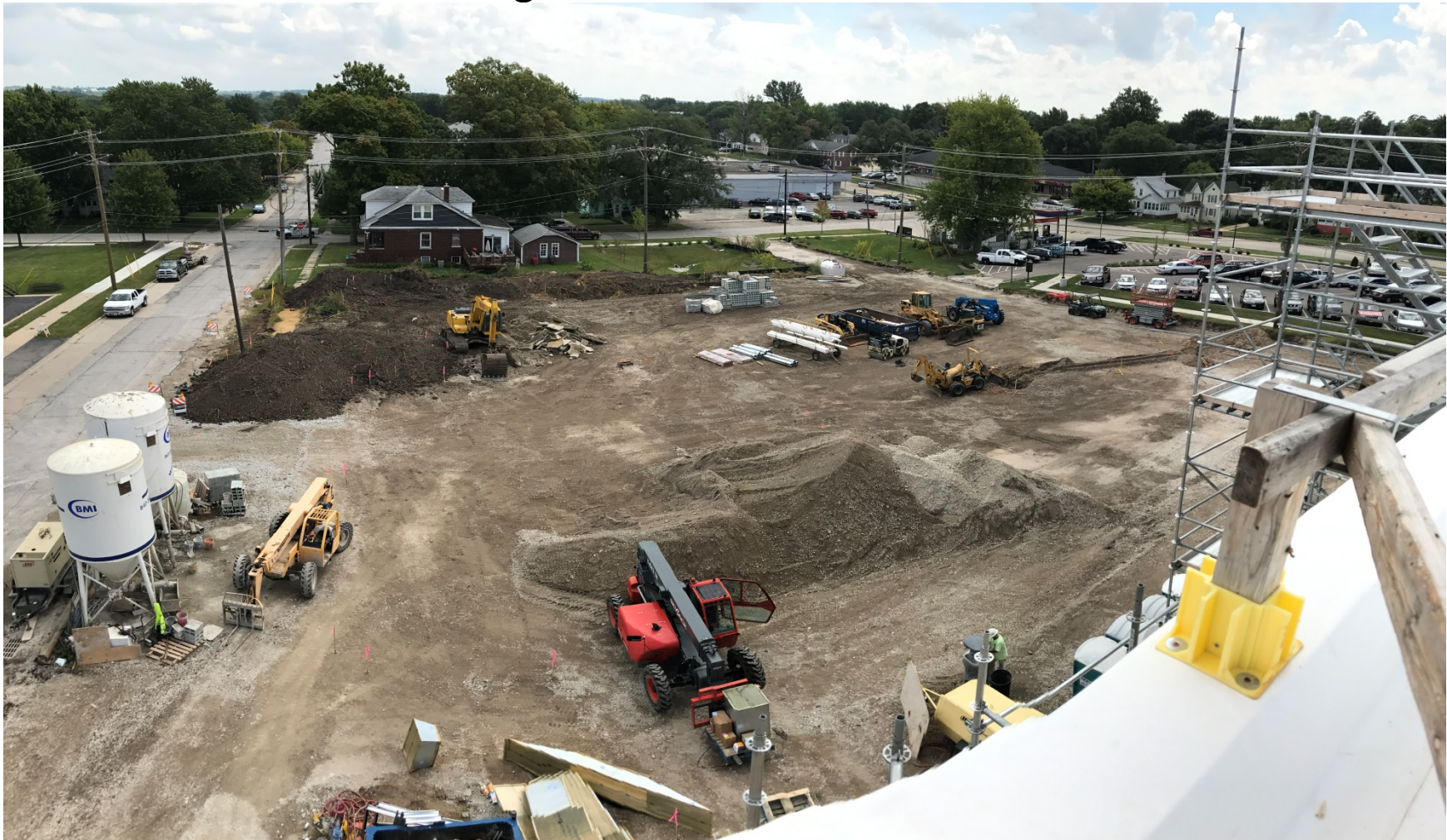
Sitework Progress in Employee Parking Area
