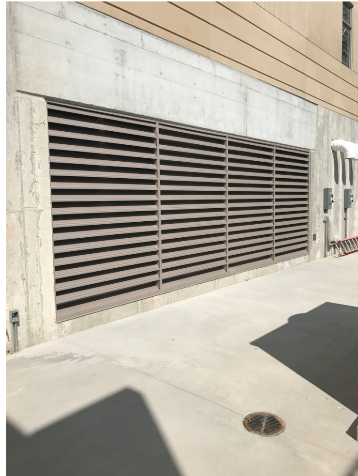
Exterior Louver & Security Bar Grille in Basement Wall
