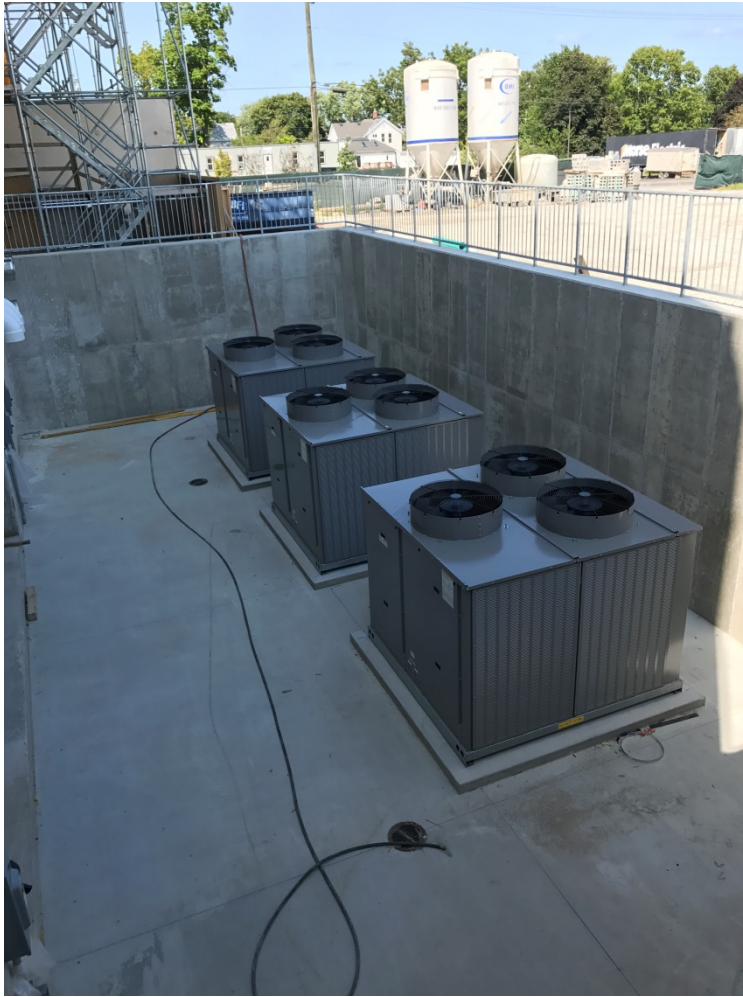
Condensing Units for AHU's (Left) and Boiler Progress (Right)
