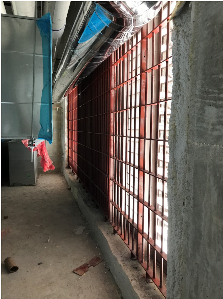
Exterior Louver & Security Bar Grille in Basement Wall
