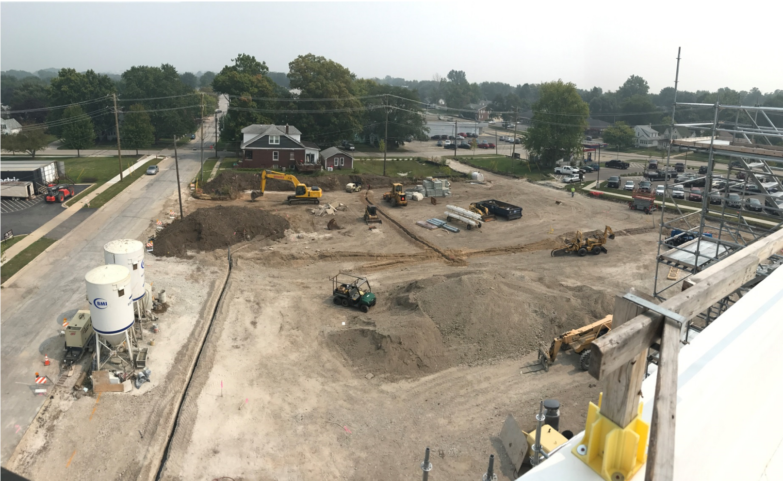
Site Progress in East Parking Area
