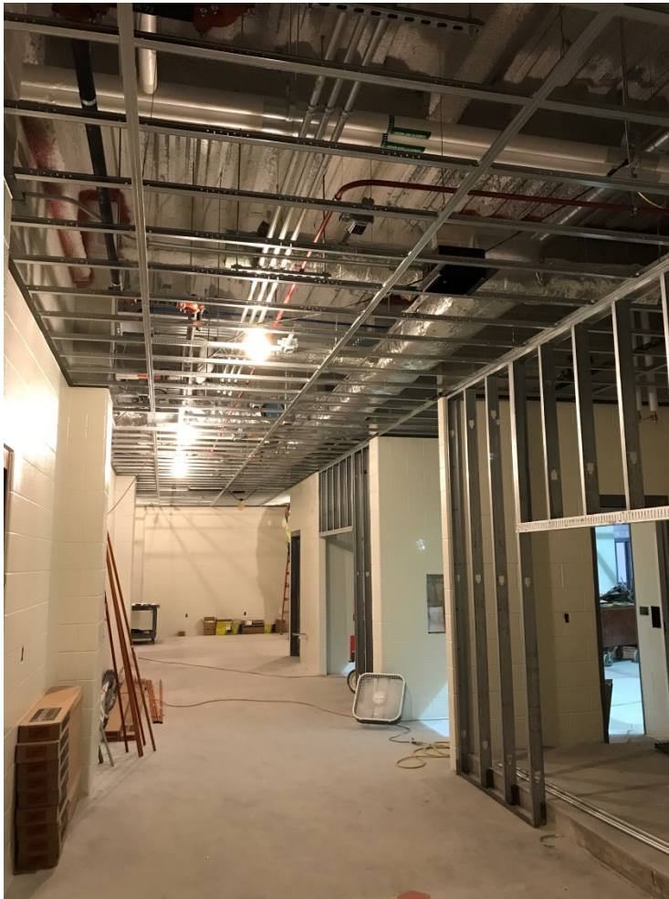
1 st Floor Kitchen Ceiling Install (Left) & 2 nd Floor Control Platform Build (Right)
